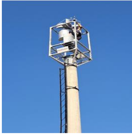
Pic 1. Installation of a wind power plant.
